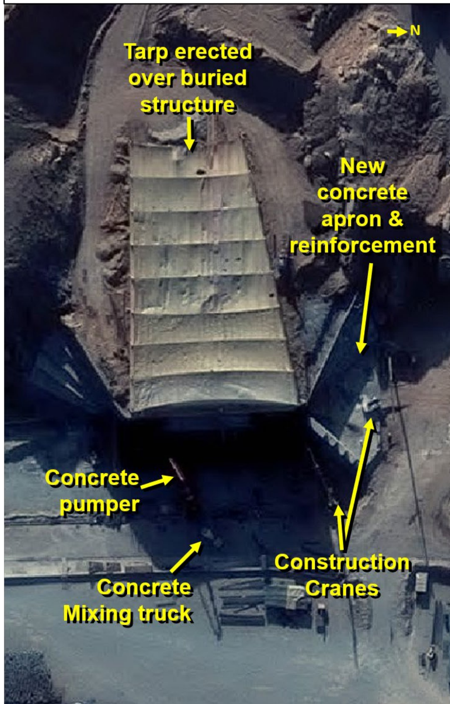
Figure 1. A close-up view of the reconstruction activities at Taleghan 2.
